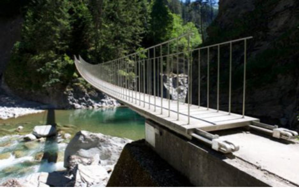
Brücke Suransuns, Viamala
